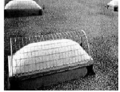
ŞEKİL 1:Kapak Sistemleri ( Montana Department of Labor and Industry Safety and Health Bureau, Fall Protection in Construction, 2010, S.35.)
